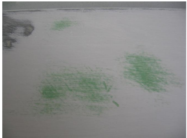
Close up view of a low spot (green) that will require more filler.
