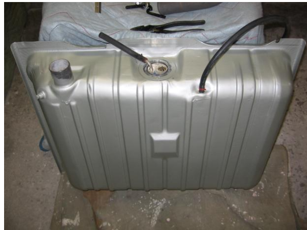
The gas tank has the fuel sender and vent hose installed prior to being lifted into place.
