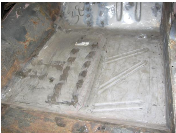
New right floor pan is in place.
