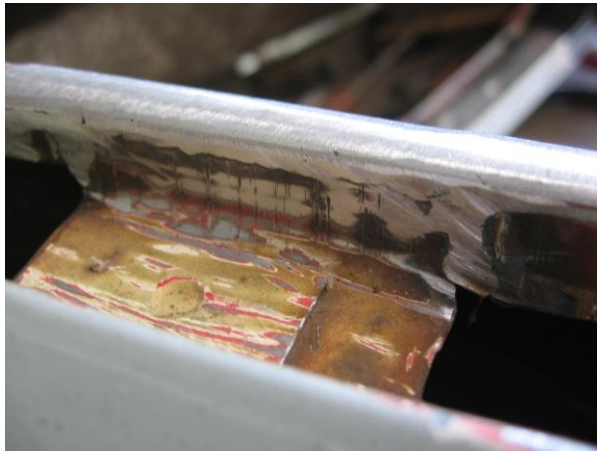
The fatigue crack is welded back together.
