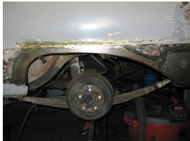
The wheel lip patch has been MIG welded into place.
