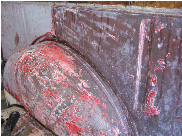
Yes, every square inch needs to be stripped including the inside surfaces.
