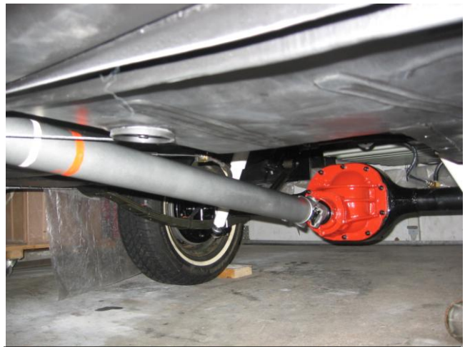
Drive shaft installed, the orange and white stripes duplicate the original factory markings.
