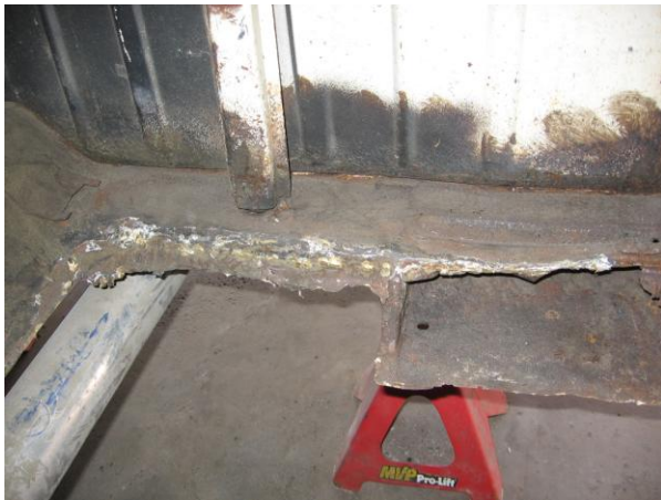
The floor patch behind the driver has been removed; if you look close you can see sealant and brazing.
