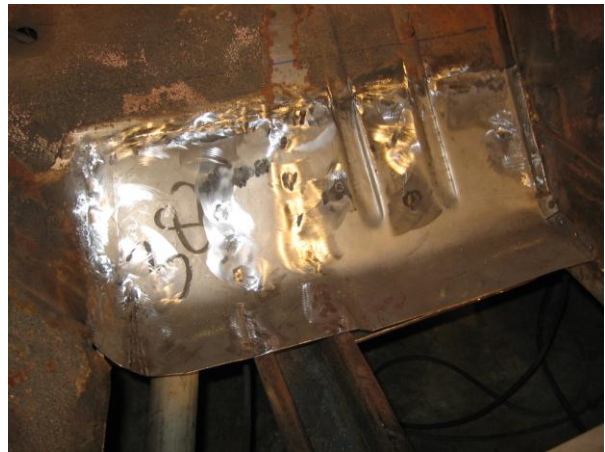
New right toe board is welded in place
