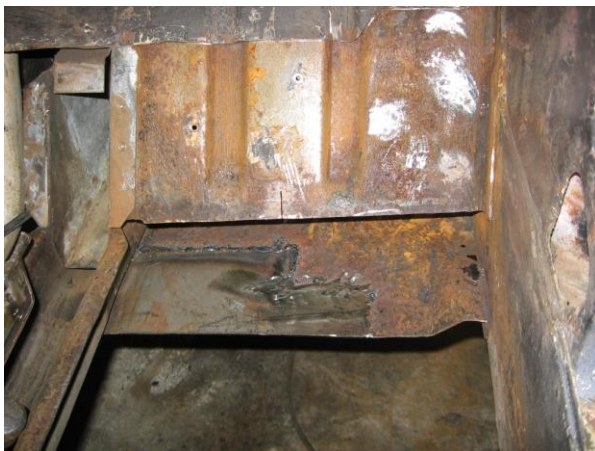
The right floor of the torque box repaired
